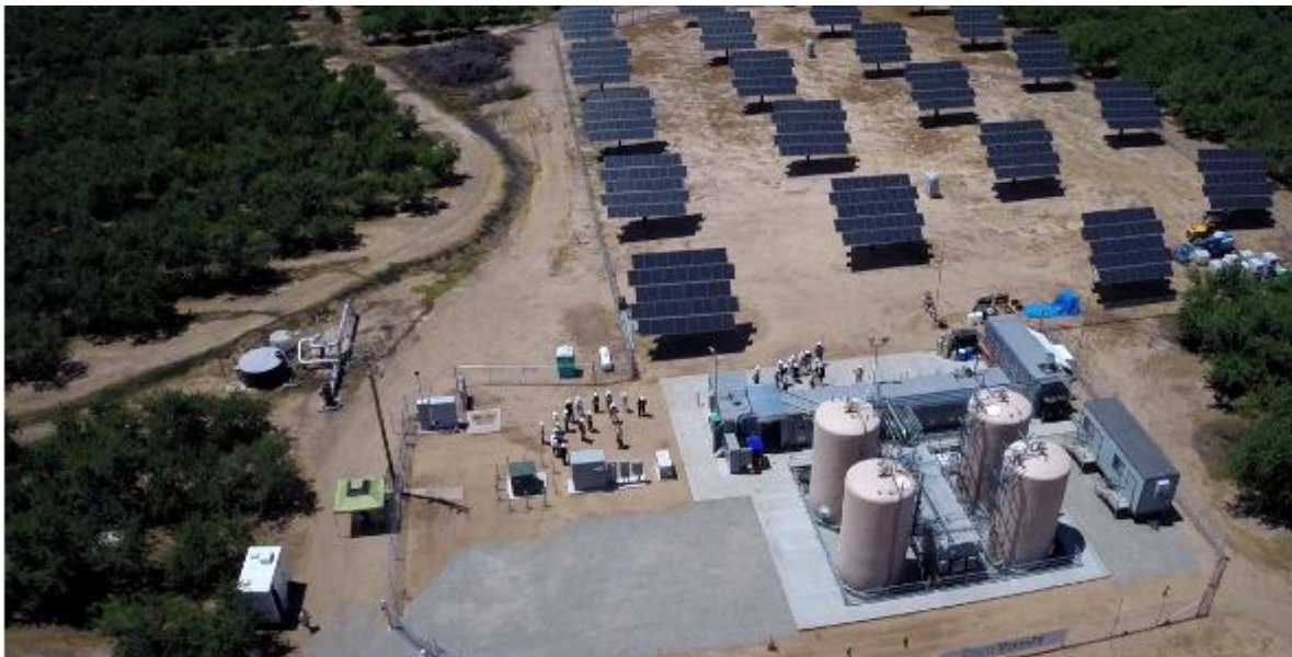
Enervault Flow Battery Installation
